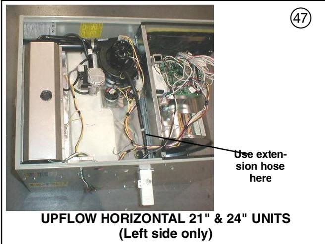
next to the secondary recuperated cell. Remove the larger drain line (from the secondary cell) and trim to fit between the secondary cell and the new trap location. On upflow units, plug the hole in the blower deck where the tube went through.
