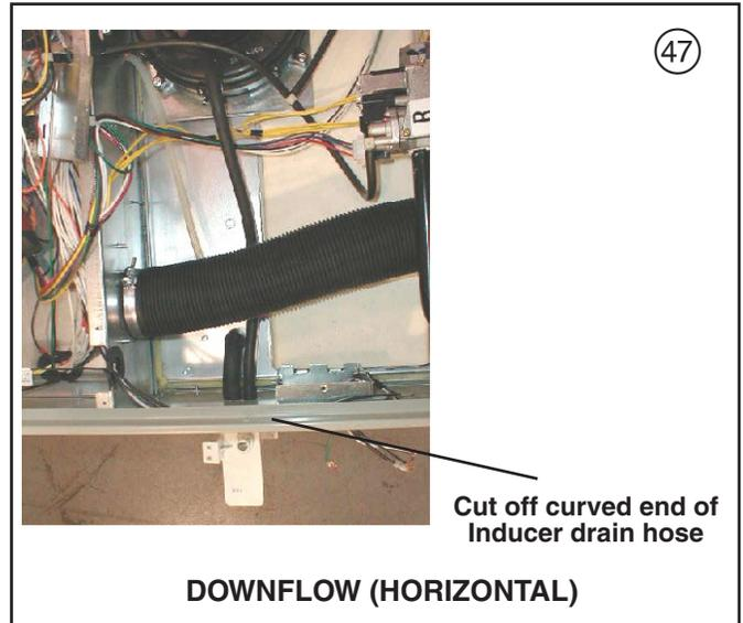
Remove the hose from the induced blower and reposition into the other drain tap of the inducer, which is located 90° clockwise around the inducer. Move the cap from that drain tap to the unused drain tap. On upflow units, plug the hole in the blower deck where the tube went through. This tube on downflow units will need to be cut to fit between the inducer and the trap. On upflow units, this tube may need to be extended, using the tubing shipped with the furnace.
